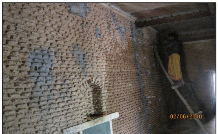
View of the internal renovation work in progress
