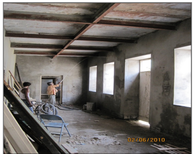
Renovation work in progress (Inside View)
