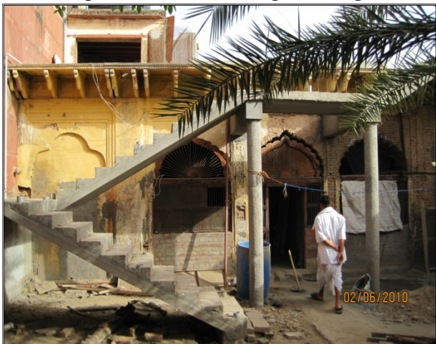
View of the new staircase
