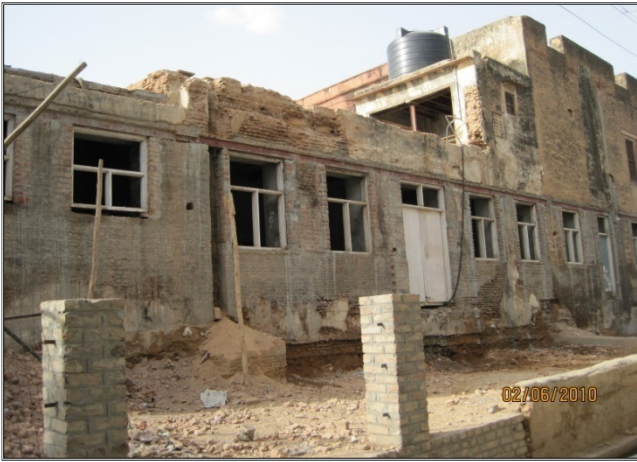
Renovation work in progress (Outside View)
